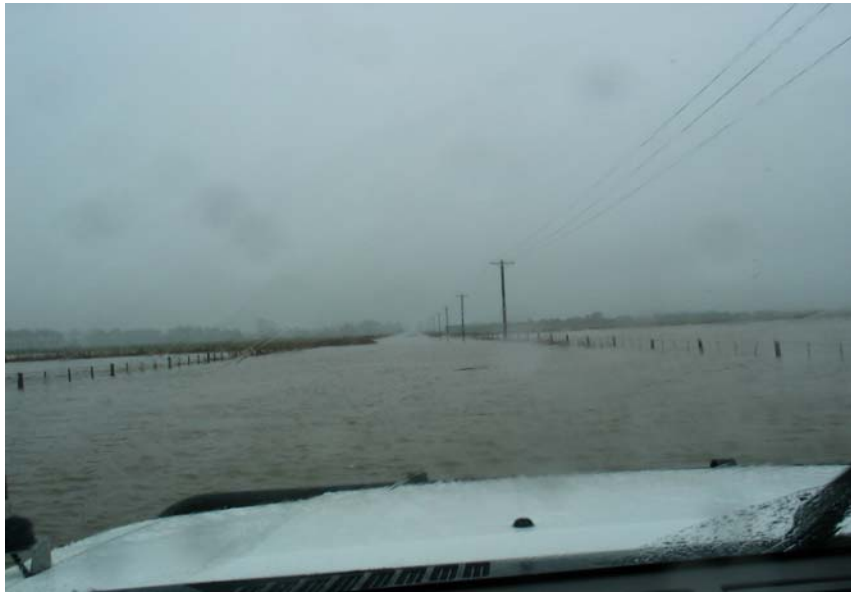
Crowes Road Flooding 31/7/07
