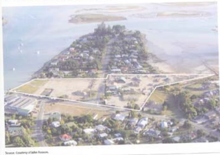
AERIAL VIEW OF THE ABANDONED FRUITGROWERS CHEMICAL COMPANY SITE AT MAPUA.
