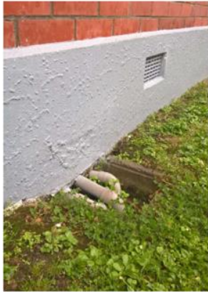
Photo 2 – Low gully trap
