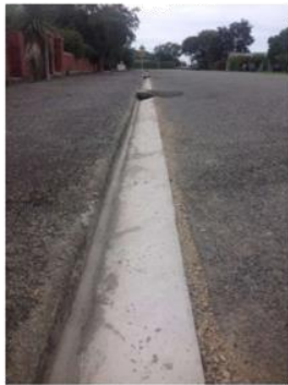
Photo 3 – Infilled deep channel
