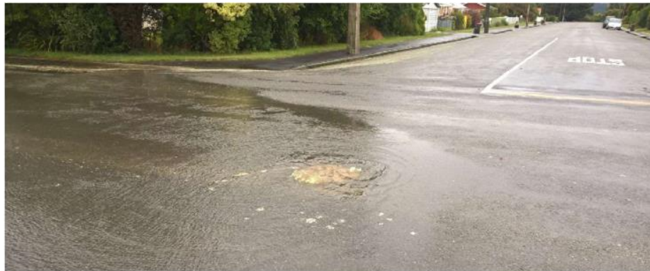
Photo 1 – Surcharged manhole corner Edward and High Streets
