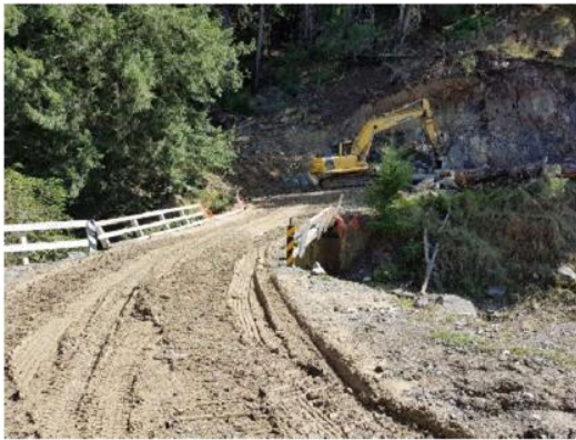
Photo 7 - Lanes Bridge on Kaiwarua Road – rock bluff removal
