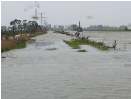
Photo 9 - Hook Swamp Road Closed due to Flooding
