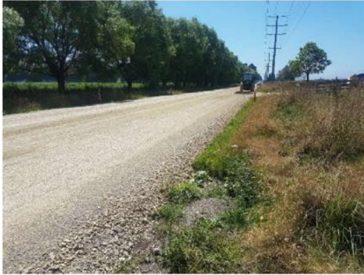
Photo 6 - Old Ferry Road Overlay before sealing
