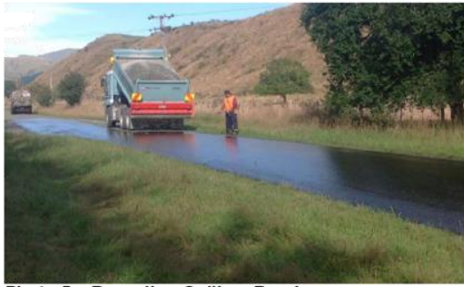
Photo 5 – Resealing Colliers Road
