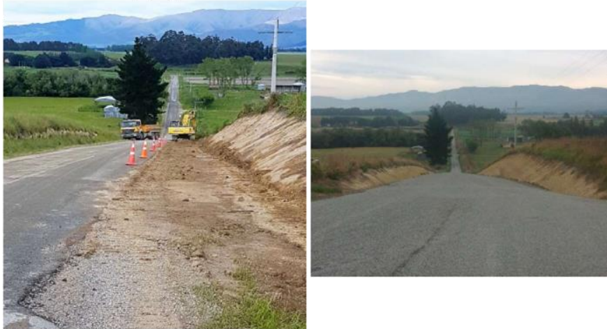
Photo 8 - Tavistock Road seal widening and reseal
