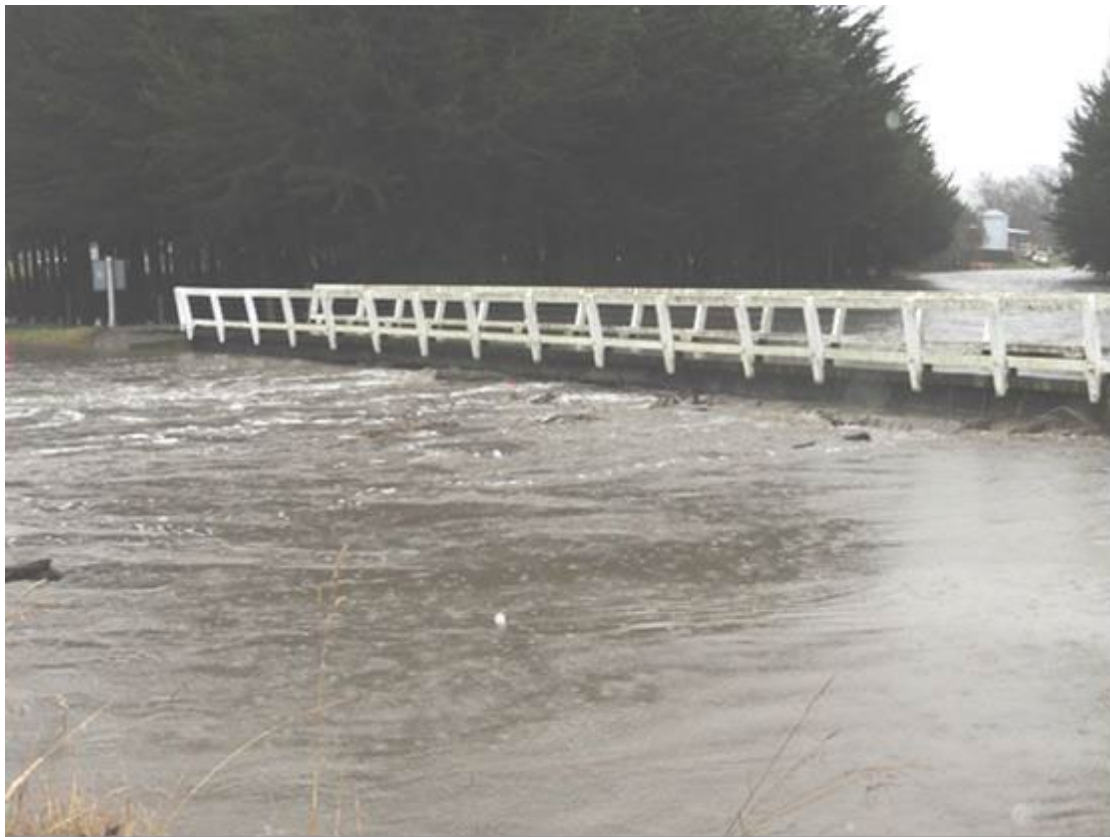
Holme Station Corner Bridge in Flood conditions
