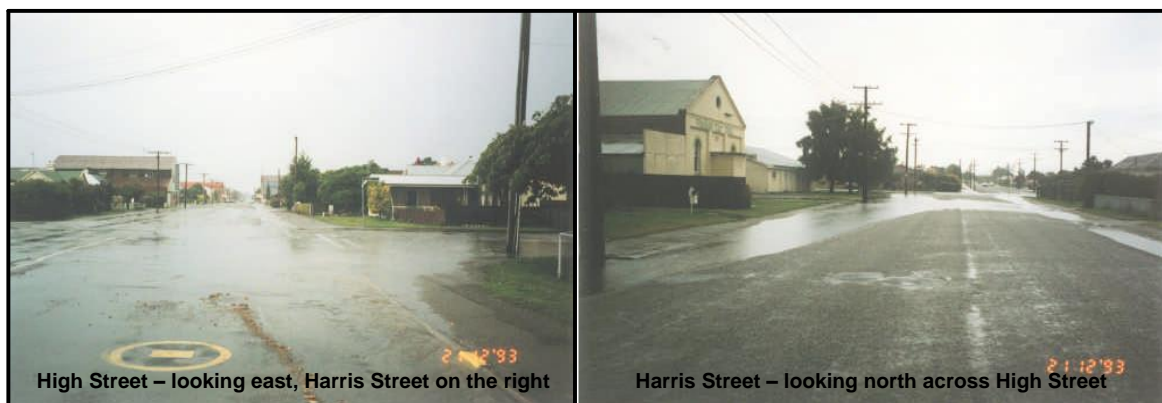
Figure 3-6: Localised street flooding prior to the 2013 upgrades
