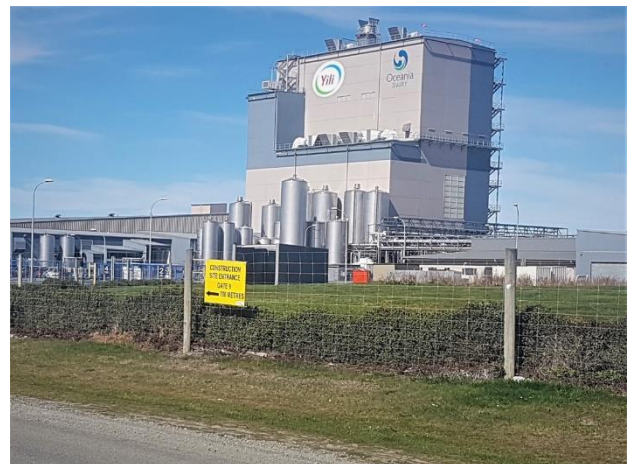
Figure 6.6 - Oceania Dairy Factory (Cooneys Road, Glenavy)
