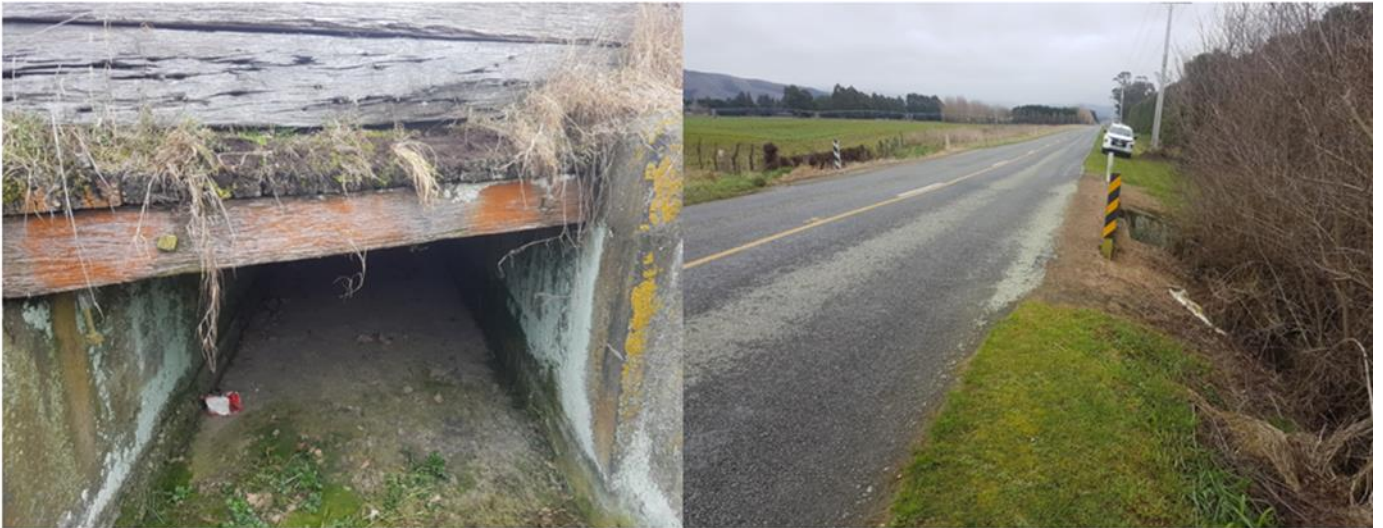
McNamaras Road Culvert Replacement
