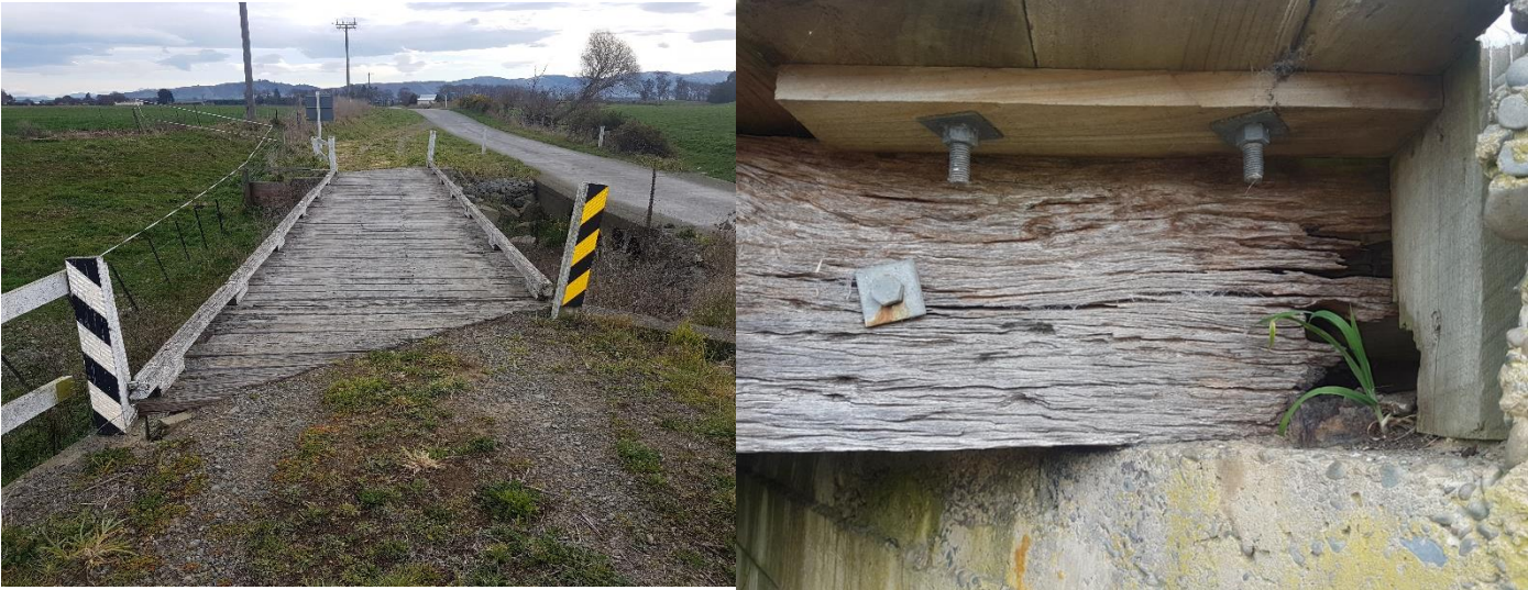
Scarletts Bridge Replace superstructure.
