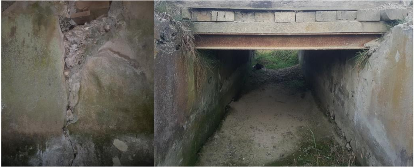
Hillboro Culvert Replacement
